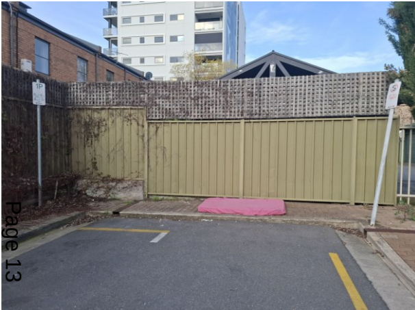
Image: Before bin surround installation
